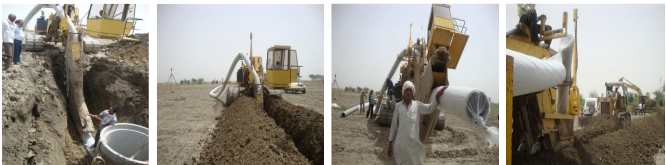
Fig. 3 Subsurface drainage machinery being used in Haryana
